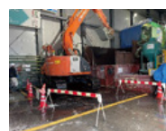
Excavation work at shield shaft
