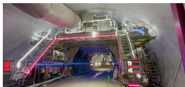
Automatic concrete-laying robot "Centring Futures"® for lining mountain tunnels
