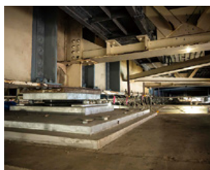
New bearing installation
