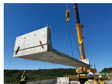
Installation of integrated deck slabs and barriers
