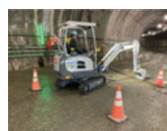
Roadbed maintenance work at tunnel entrance
