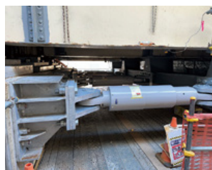
Cold-weather specification seismic dampers
