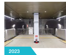
2023 Sotetsu-Tokyu Direct Line Tsunashima Tunnel
