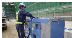
Refueling a generator at a construction site
