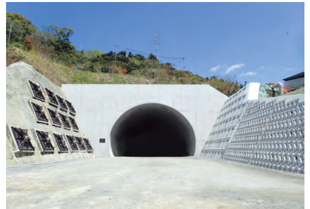
Arida Kainan Road No. 5 Tunnel construction
