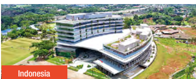
Indonesia Knowledge Hub Construction: S-RC Scale: 8 stories above ground Floor area: 67,112 m 2 Use: Office building
