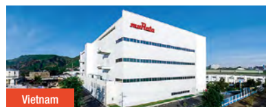
Vietnam Danang Murata Construction: RC Scale: 4 stories above ground Floor area: 26,754.17 m 2 Use: Factory (small electric component manufacturing plant)
