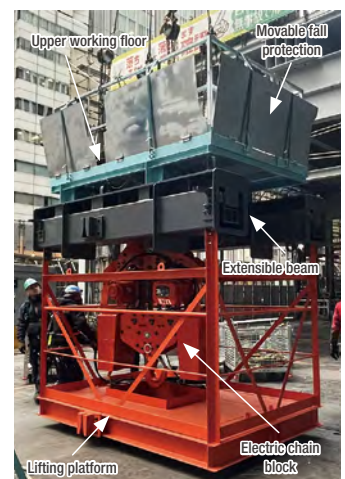
Working floor and lifting unit
