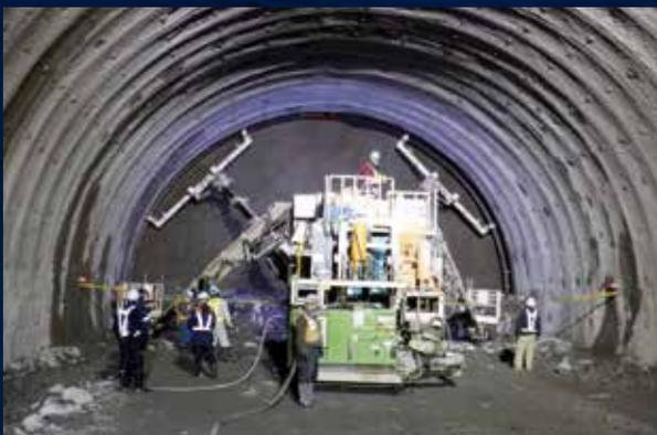
Unmanned Tunnel Face Construction System
