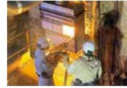
Construction Work in Progress (Cutting a Retaining Wall)
