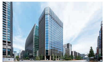
Construction of Nittetsu Nihonbashi Building Nippon Steel Kowa Real Estate Co., Ltd.
