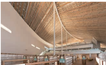
Construction of Nagasaki Pref. & Omura City Library, Omura City History Museum Omura City, Nagasaki Prefecture
