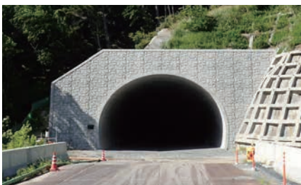
Construction of Chubu-Odan Expressway Kamiyagisawa Tunnel
