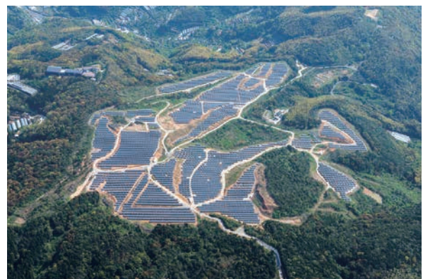
Nagasaki Tadewara Mega Solar Power Plant
