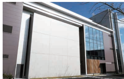
Structural and construction laboratory building (scheduled completion in November 2019)
