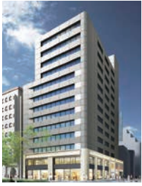
Acquisition of the Toda Building Shinsaibashi (after renovation)
