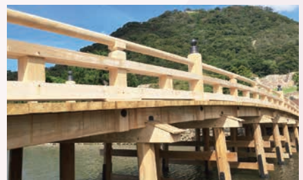
Restoration works of Tottori Castle Remains Giboshi Bridge
