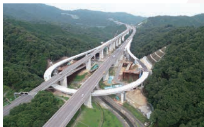
Construction at Shin-Meishin Expressway Kameyama Nishi Junction Ramp (substructure)
