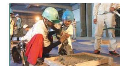
Parent and child experience construction with concrete
