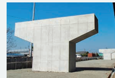
Yamoto Ishinomaki Highway substructure construction Tohoku Regional Development Bureau, Ministry of Land, Infrastructure, Transport and Tourism
