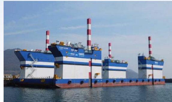
Semi-submersible barge FLOAT RAISER (Hataage)
