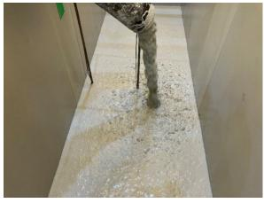
Picture 1: Outlet poring Carbon Negative concrete
