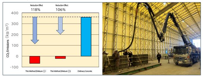
Figure 1 CO<sub>2</sub> Reduction Effect of Carbon-negative concrete 32 and Photo showing pouring concrete
