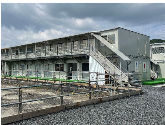
Photo 1: ZEB-certified field office
